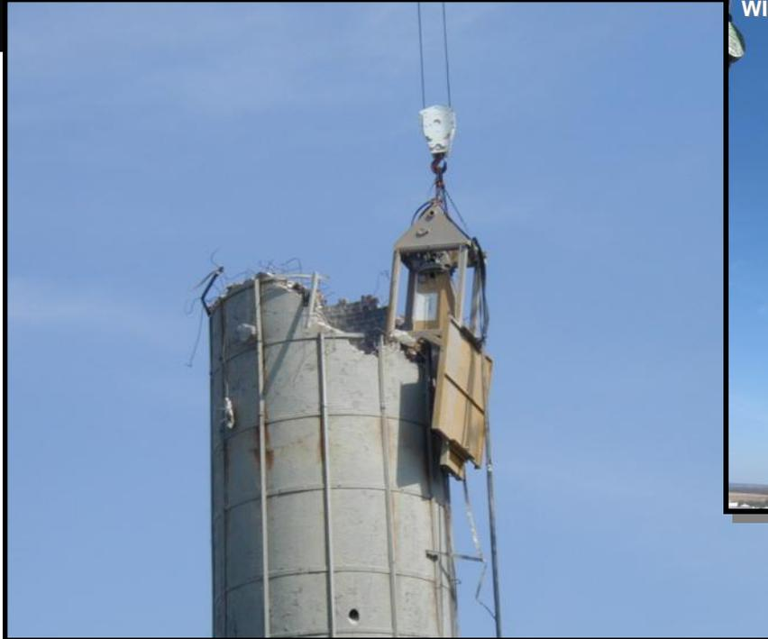
CRUSHER UNIT BEING LIFTED WITH CRANE TO STACK TOP
