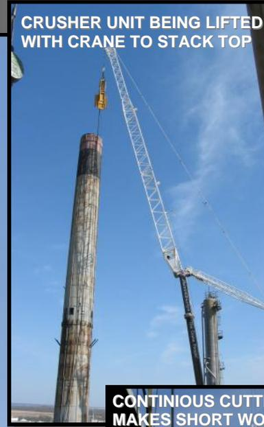
CONTINUOUS CUTTING ACTION MAKES SHORT WORK OF TALL STACKS
