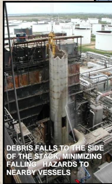
DEBRIS FALLS TO THE SIDE OF THE STACK, MINIMIZING FALLING HAZARDS TO NEARBY VESSELS
