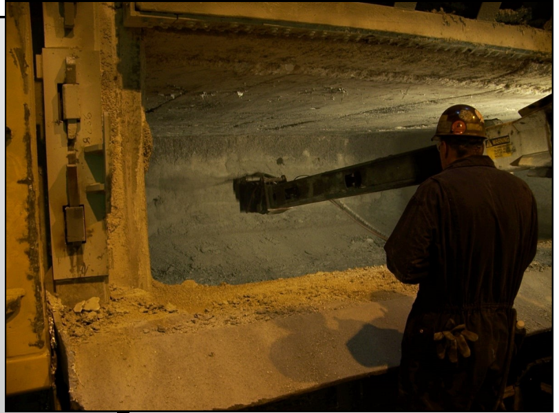
KT-30R Applying gunnite to the back wall
